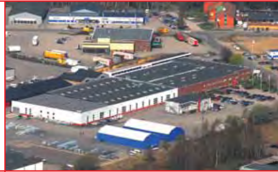
IV Produkt's head office and production facilities are situated in Växjö, Sweden. The company is owned by IV Produkt Holding AB.
