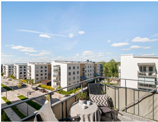
Flats in Stockholm, Sweden
